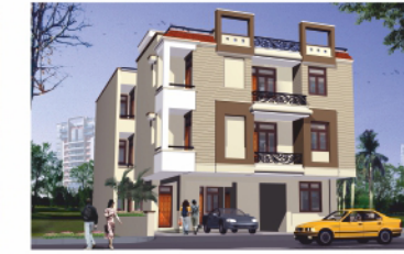
Aastha Apartments, Nirman Nagar
